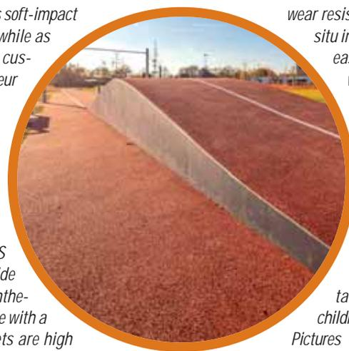
wear resistance and low maintenance costs. The seamless in-situ installation method allows the two-course surface to be easily installed on undulating and angled substrates as well. The undulating substructure in Heidelberg consists of pervious concrete and steel plates for lateral stabilization.
